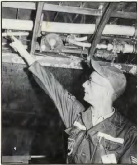
S/Sgt Jones points to a newly treated fuel line in KB-50 flap well area.
