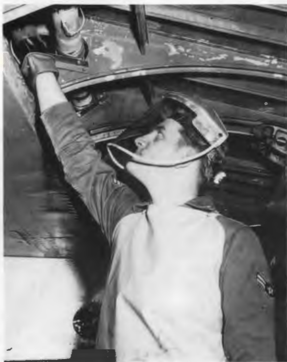
Airman Morris treats a fuel line in the KB-50 flap well area. Many of the treatment processes require painstaking hand labor.
