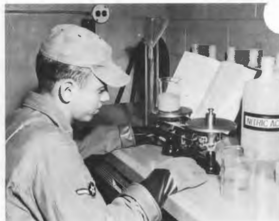
Airman Britner mixes a chromic pickle solution to treat magnesium. Cleaning solutions are strong, and make rubber gloves and other protection necessary.
